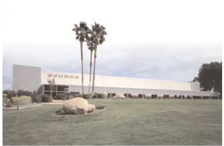
Bourns Corporate headquarters in Riverside, California
