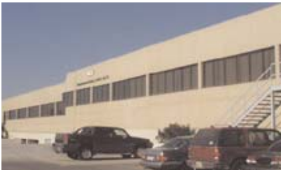
BCLM production facility
