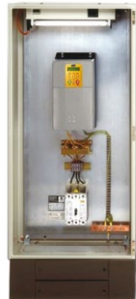
DC590+ DRV equivalent illustrating panel space saving
