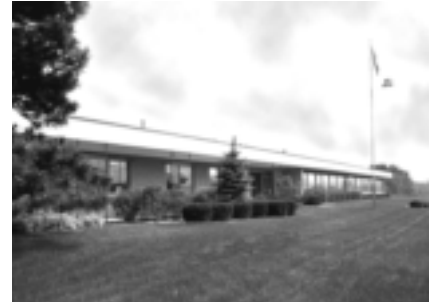
USA – Danaher Controls Gurnee, Illinois
