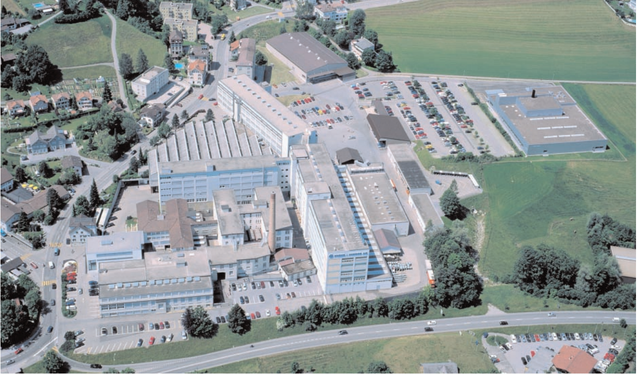
Plant in Herisau
